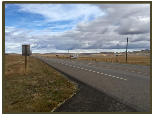
Figure 7. Highway 287, north of the I-90 Interchange
